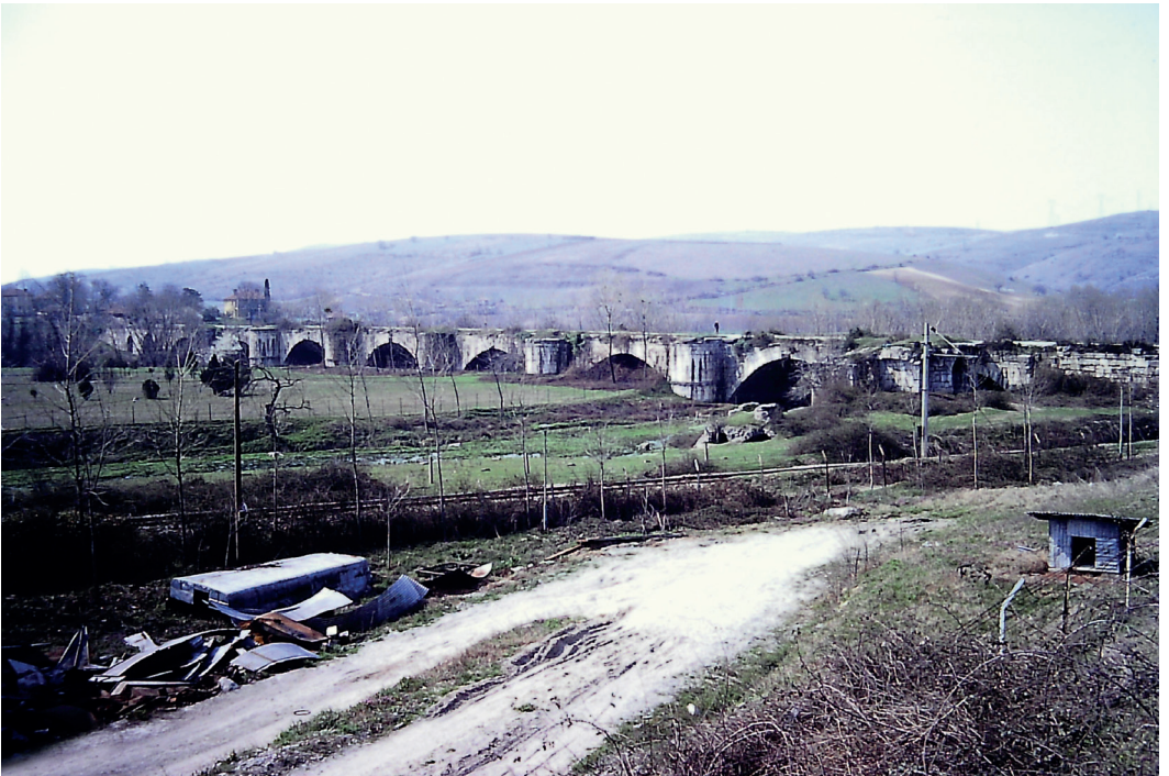
Justinian's Bridge over the Sangarius. (Author)
